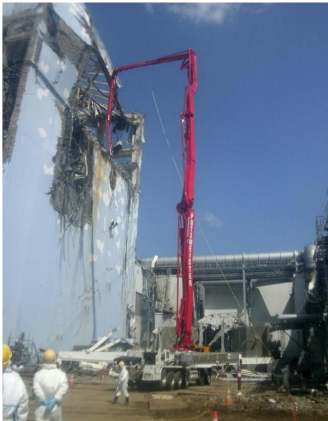
Figure 1: A concrete pump injects water into the spent fuel pool of the severely damaged Unit 4 of the Fukushima Daiichi nuclear power plant. (Photograph: TEPCO)
